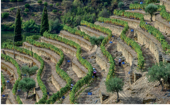
THE 'PORT ARTHUR' STONE TERRACES AT QUINTA DOS MALVEDOS
